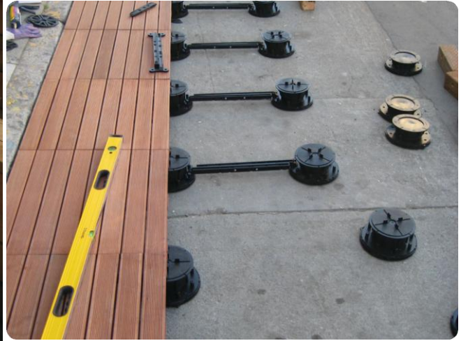
Bison pedestals are a popular substructure for parklets.
